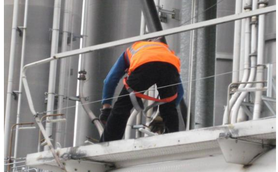
Harness not fitted correctly
