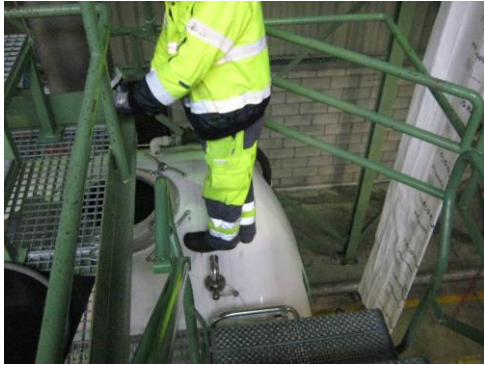
Fall restraint system not properly designed / Gaps which allow a worker to fall through
